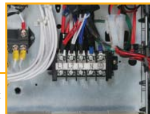
Outdoor unit power supply terminal block
