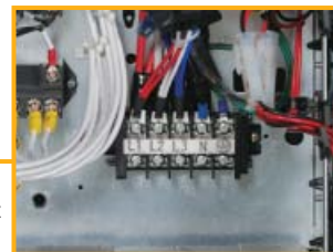
Outdoor unit power supply terminal block
