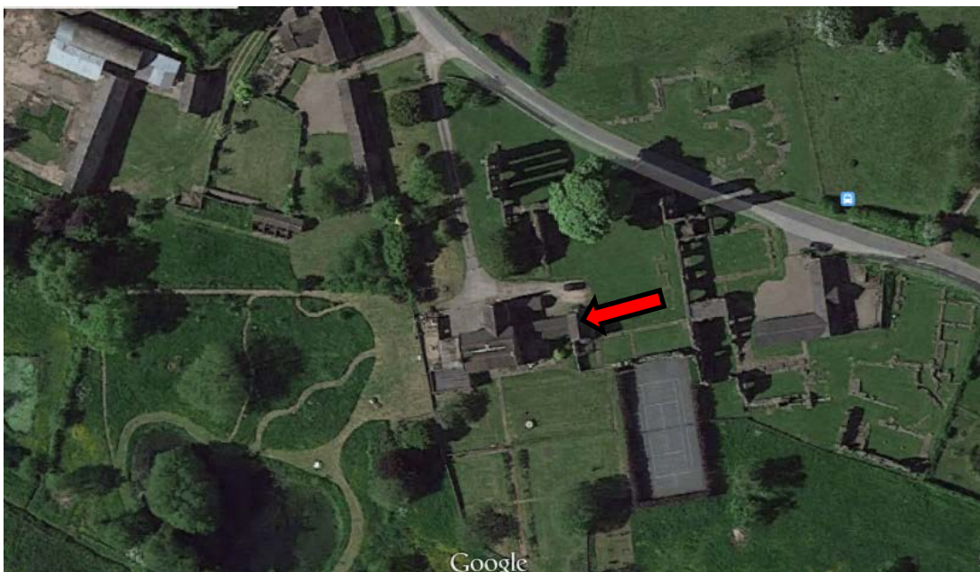
Image 7.0: Granary and Linking Service Wing
