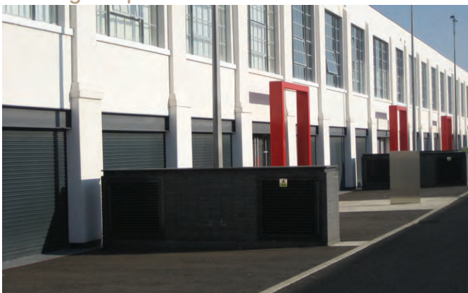
↑ The red detailing breaks down the frontages and marks the entrances
