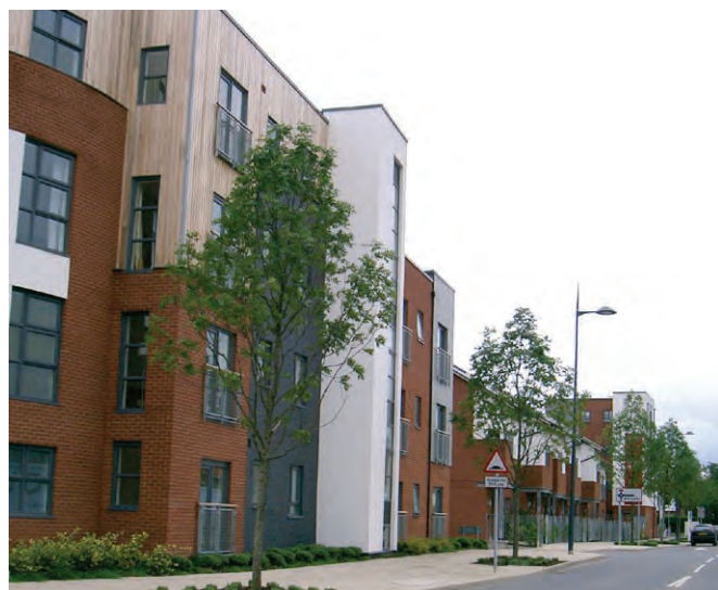
Wider street with avenue planting at Didsbury Point in Manchester
