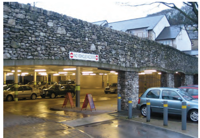
↑ Underground parking takes advantage of change in levels to hide parking and maximise use of a site
