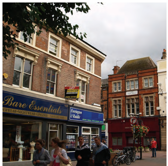
Burton-Upon-Trent town centre includes a mix of different land uses
