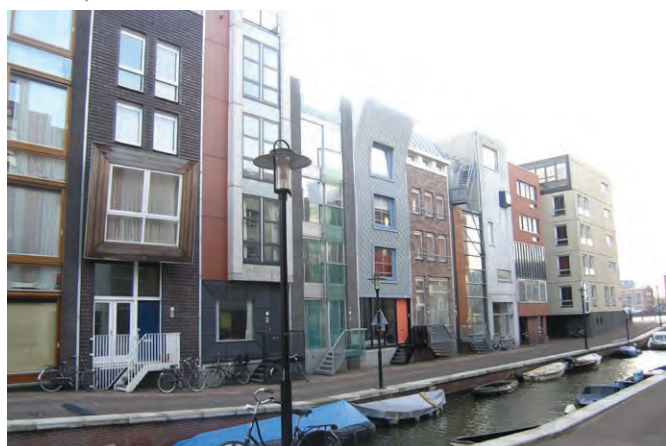
↑ Consistent height and width to building plots unites varied contemporary architecture
