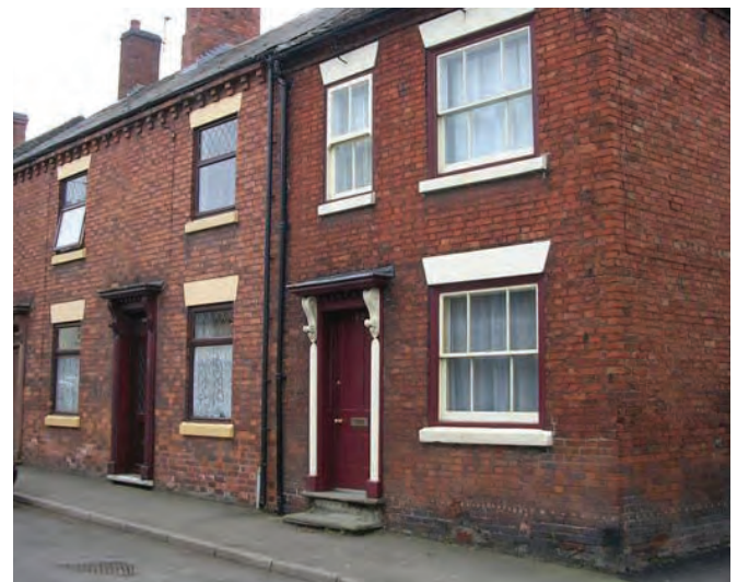
↑ LEFT: Inappropriate alterations RIGHT: sash detailing
