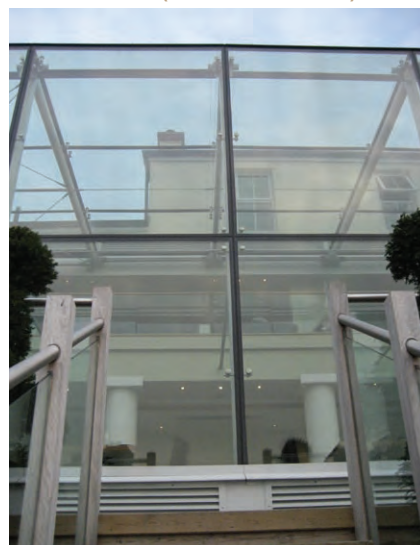
↑ A sensitive but striking contemporary extension adds to the quality of the original building
