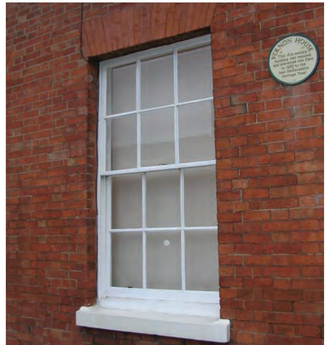
↑ An original sash window with sill and lintel
