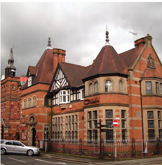
This building turns the corner effectively creating a local landmark
