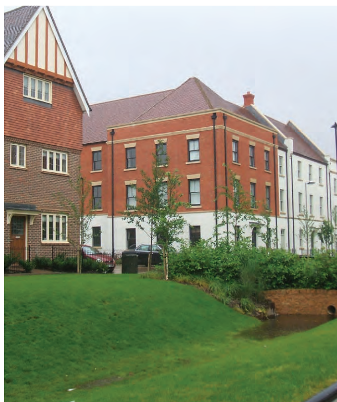
↑ Sustainable Drainage at Upton Northants
