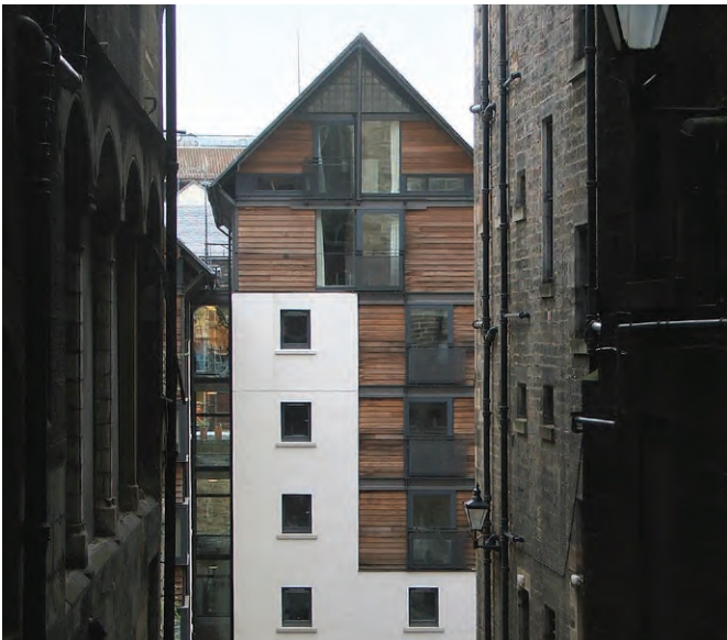
The gable is aligned to terminate the view/vista along the street
