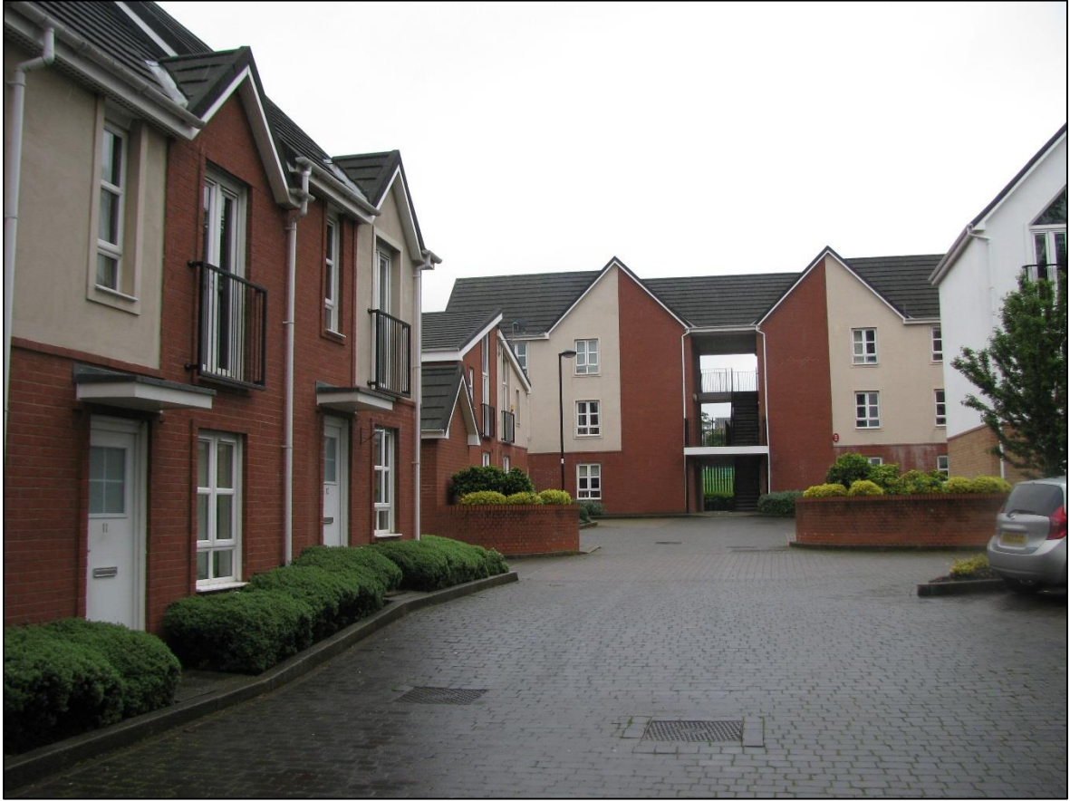
High quality residential development within Stapenhill
