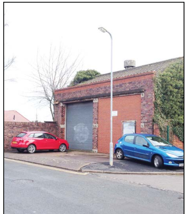
Potential brownfield site, Cockstubbles
