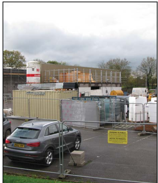
The Leisure Centre during renovation in 2015
