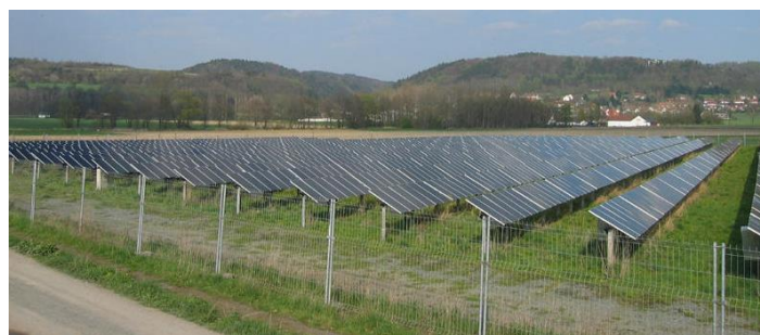
Figure 2. Module tables oriented towards the south.
