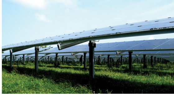
Figure 3. Lower border of module table 80 cm above the ground.
