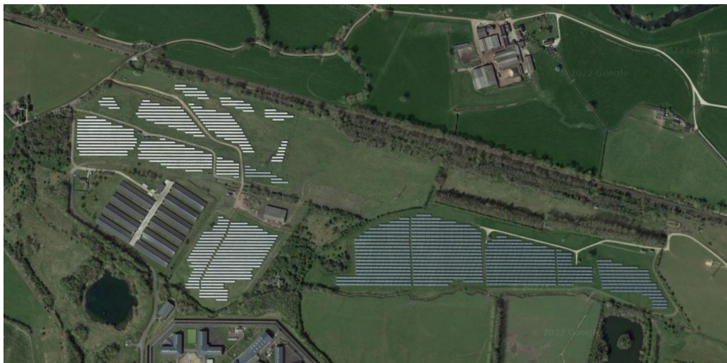
Figure 3: Google Maps image of Green Lane and Moat Farm Solar Farms
