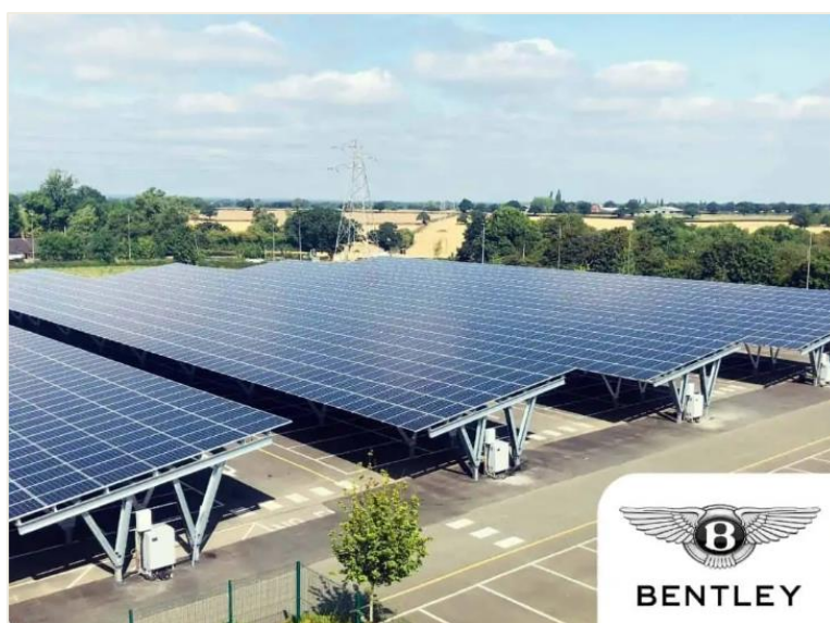
Figure 2: Solar Car Park at Bentley Stoke on Trent
