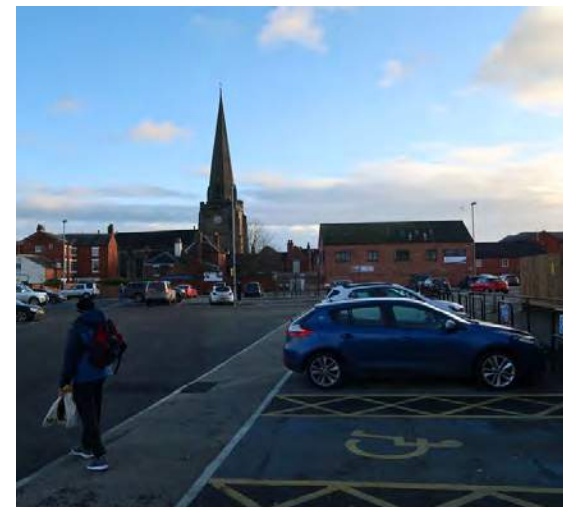
View from the Maltings car park looking south-east towards the Parish Church of St Mary (Grade II* Listed)
