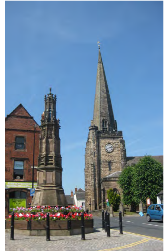
View the Market Place looking north towards the Uttoxeter War Memorial (Grade II Listed) in the foreground and Parish Church of St Mary (Grade II* Listed) set further to north
