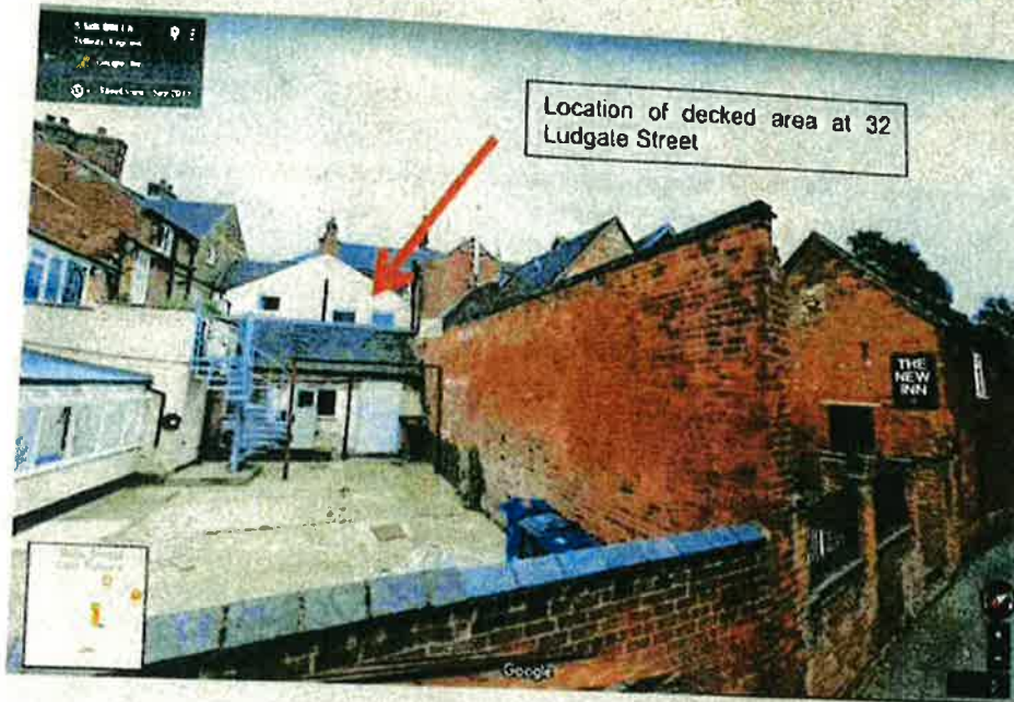
Image of rear of New Inn adjoining wall to 32 Ludgate Street
