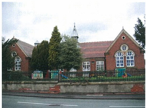
The Thomas Russell Infant School, is a positive building within the conservation area.
