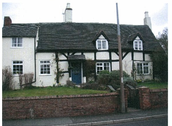
One of the several timber framed buildings within the conservation area.
