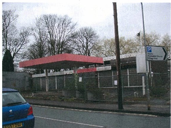
Derelict garage site detracts from the aesthetic quality of the conservation area
