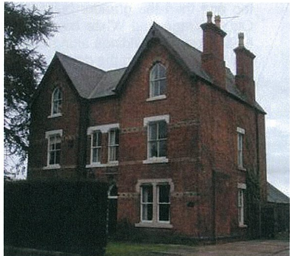
Victorian semidetached houses to the south of Station Road.
