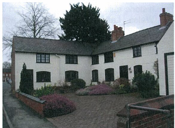
Listed building 25, 25a and 27 Wales Lane of early 19 th century date
