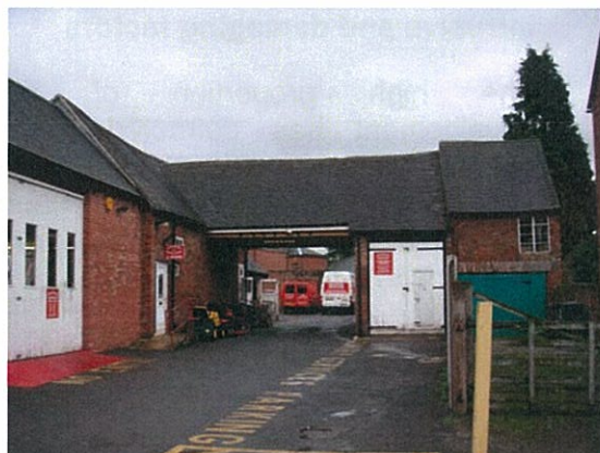
Reused building on Bell Lane, with redbrick and timber detailing
