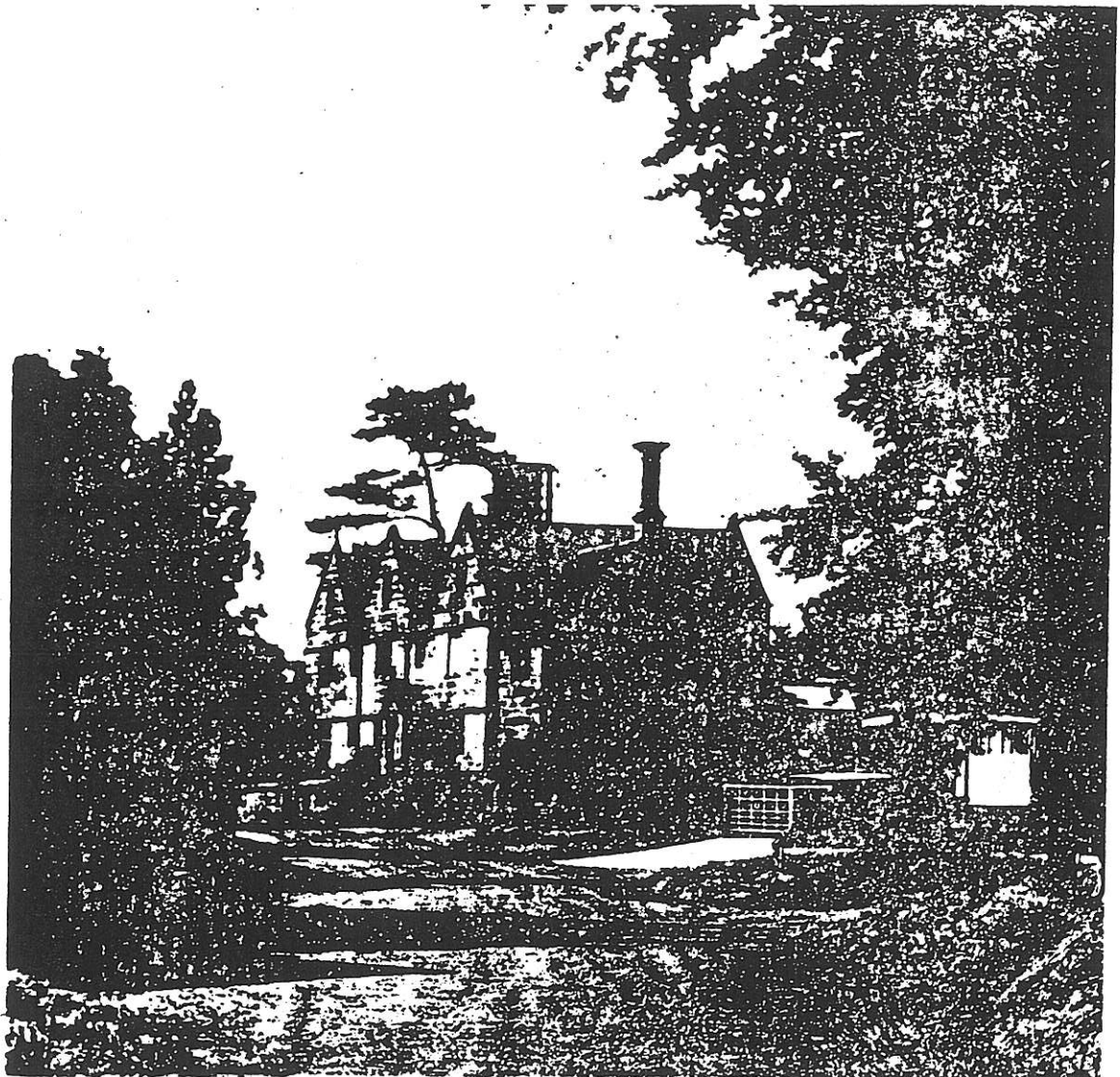
Old Hall Farm House
