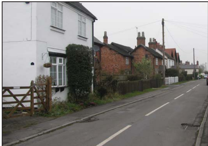
Tarmac is used widely in the public realm
