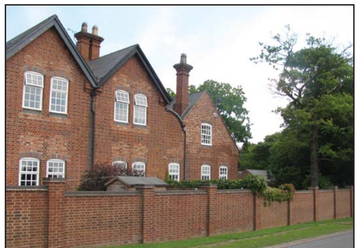
Red brick is the dominant building material
