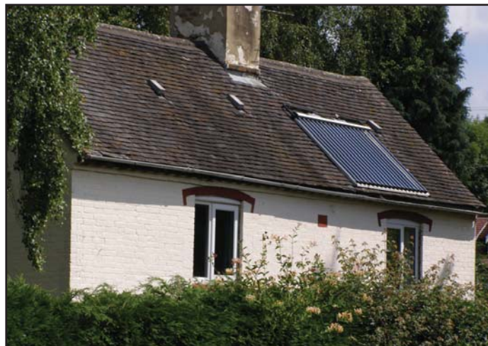
Solar panels detract from the special designation
