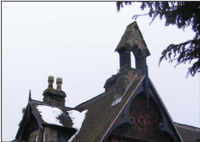
The now redundant bell tower at All Saints School
