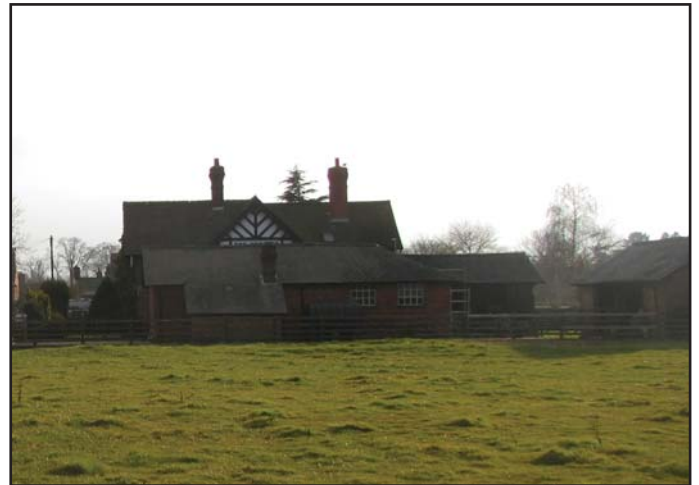
Forest Gate Farm, Chapel Lane
