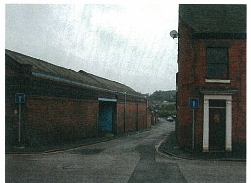
11: The former Leighton Ironworks off Pinfold Street
