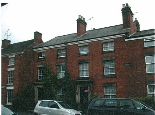
5: 33-39 Balance Street – three storeyed 19 th century artisans’ dwellings
