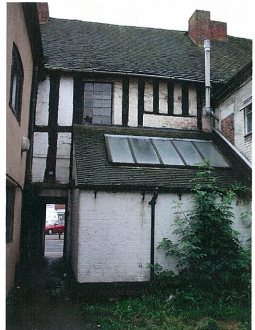
9: Medieval timber framing exposed to the rear of 32 Market Place
