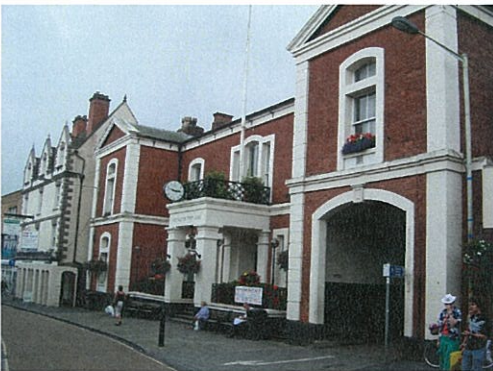
1: Uttoxeter's Town Hall and the former Cross Keys Hotel beyond
