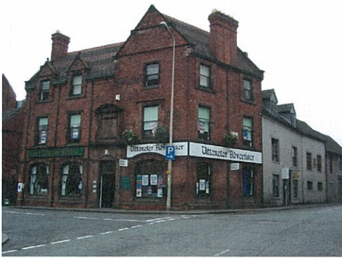
17: The Uttoxeter Advertiser building at the north east corner of the Market Place - a well-detailed solid building in dark red brick and with a fine tiled roof covering and decorative ridge. This building occupies a key site and provides a focal point at the head of the Bridge Street approach to the Conservation Area. It should be locally listed.
