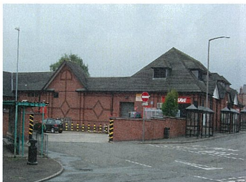
46: The uninspired architecture of the former Kwik Save supermarket (now the Co-op), with its derivative and empty motifs and decoration does little to improve the character of the Maltings zone in this crucial part of the Conservation Area
