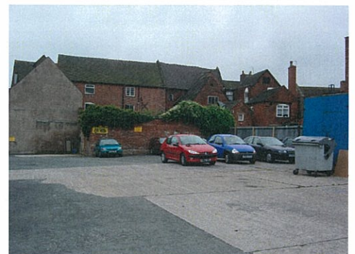
36: Lion's Buildings' parking and the rear of Market Place buildings in 2004 - a void at the heart of the Conservation Area and this zone which leaches life and character
