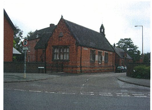
22: Clustered buildings (some listed, some not) forming part of the Alleyne's Grammar School complex
