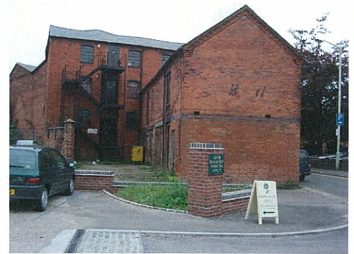
35: The Old Mill building - the key structure and focus in the south western section of Church Street
