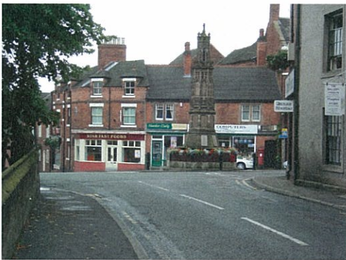
41: Low rise Victorian buildings of considerable townscape value at the northern end of Bridge Street
