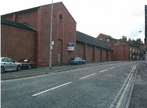
42: The traumatic impact of a poorly designed and planned modern structure on the Conservation Area (2004)
