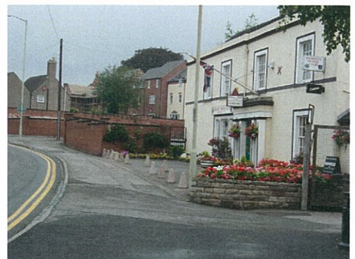
23: The Bradley House Club - harsh hard landscaping and the squat concrete bollards make a negative contribution to the overall character of the site despite its Grade II listing
