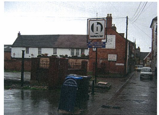
61: The barren and aggressively degrading environs to Trinity Walk in the centre of Queen Street
