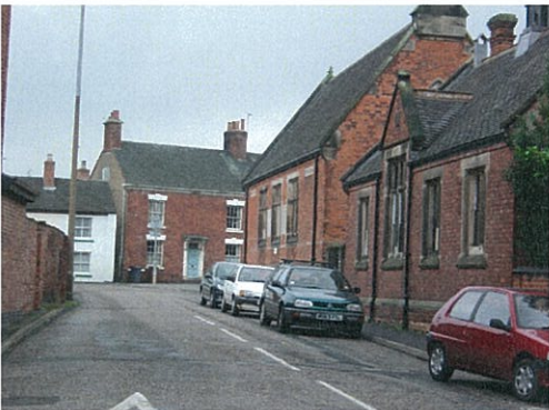
25: The view westwards along Back Lane
