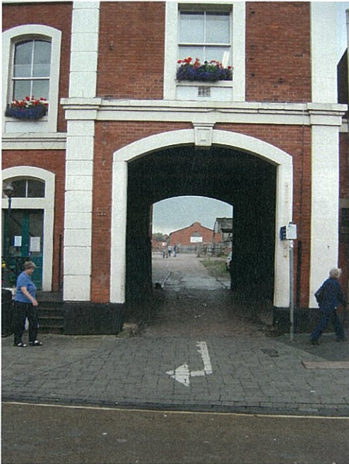
50: A glimpse of the former now-demolished Cattle Market from the High Street - an important part of the character of the town and an evocative historical juxtaposition that has been lost (but in so doing has opened up major potential for redevelopment)
