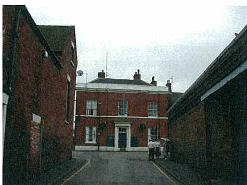
75: The listed Police Station (32 Balance Street) - architecturally interesting and providing perfect closure to the vista up Pinfold Street
