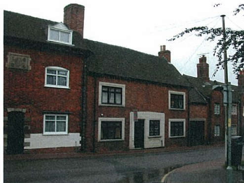
81: The former George & Dragon (65 Carter Street) - warrants local listing for its architectural interest and contribution to the streetscape
