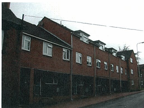
82: Jubilee Court - architecturally undistinguished and damaging to the character of this part of the Conservation Area
