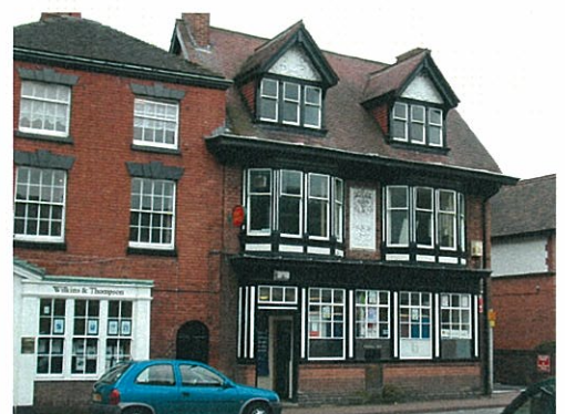
85: 15 Carter Street (Stanley House) - a strong candidate for local listing for its architectural interest and contribution to the streetscape
