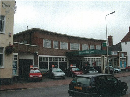
86: Sheard's Garage - architecturally important and, despite its somewhat perverse juxtaposition to the substantially greater massing of the White Hart Hotel, a serious candidate for statutory listing at Grade II
