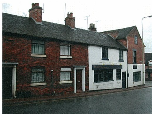
79: 75 and 77 Carter Street - typical buildings at this entrance to the Conservation Area
