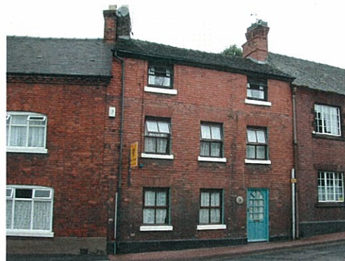
80: 92 Carter Street - a three storey artisan's dwelling - worthy of local listing for its contribution to the general street scene, as are adjoining buildings
