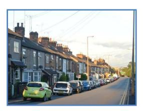
These photographs show the westerly route into Burton-on Trent. The road has a narrow width, bends and alternating gradient which is inadequate for heavy goods vehicles and further potential development in this area. Cars are parked on the pavements to reduce the risk of collision, thus reducing the pavement width to pedestrians. This is made worse on refuse collection days when pedestrians cannot walk down the pavement due to bins being left out.
